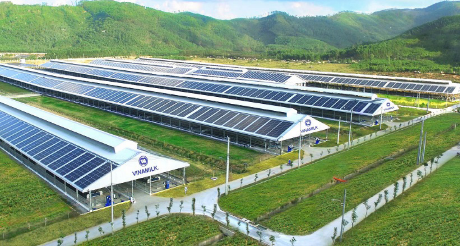
Solar rooftop at Vinamilk dairy farm in Quang Ngai.
